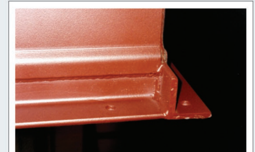
Overlapping side wall joint connections
