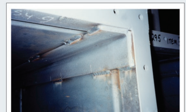
Internal heavy duty reinforcing angles
