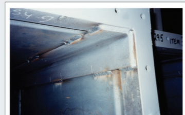
Internal heavy duty reinforcing angles
