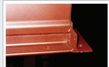
Overlapping side wall joint connections
